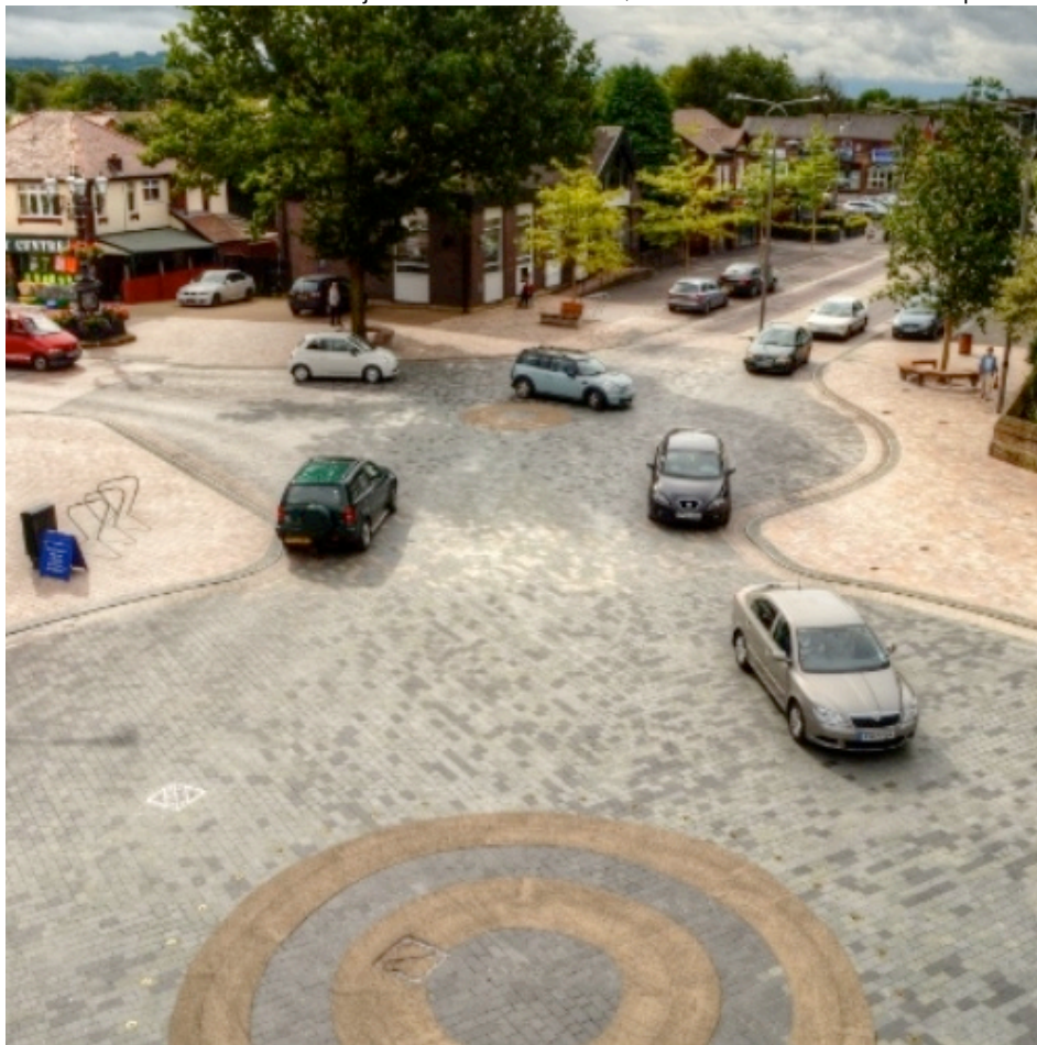
Fig. 2 Poynton, Stockport: The main junction with external controls (traffic signals) removed allowing people driving, cycling and walking to negotiate their way safely through the improved environment.
